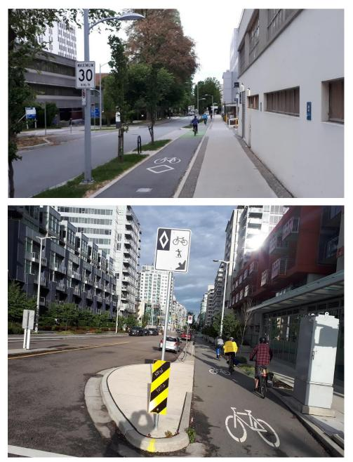
Examples of protected bike facilities in Vancouver that meet the ultimate standard. A sidewalk level protected bike lane (top) shows the bike lane separated from the road by a vertical curb and buffer.
