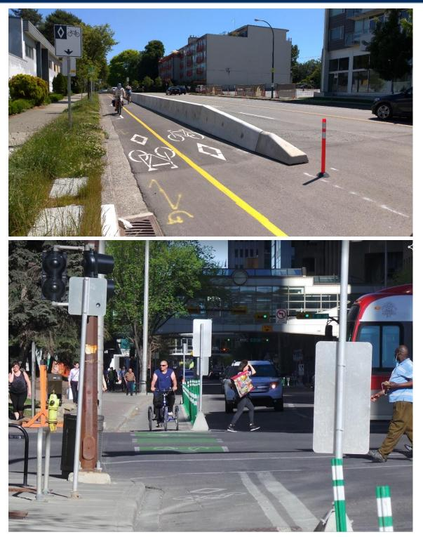
More examples of quick-build cycling facilities with a concrete jersey barrier in Vancouver (top) and flexible delineator posts in Calgary (bottom).
